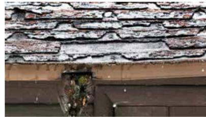
Another sign of deteriorating shingles becomes apparent when cleaning out your gutters. If you find large amounts of asphalt particles and debris in your gutters or around the perimeter of your house your roof may be starting to fail.
